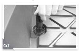
Secure fitting in position with the nut, which is applied to the underside of the tray.
