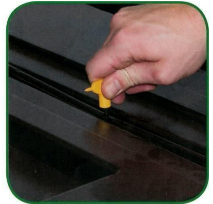
Using the holer puncher fit the connection nozzles into pierced holes
