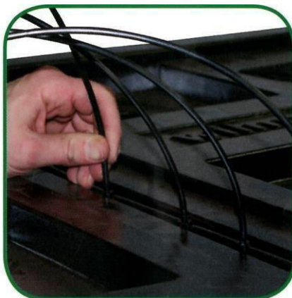
Continue to fit all Cobra hosing to nozzles along the piping
